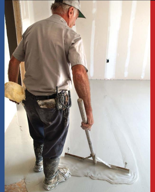
LEVELROCK<sup>®</sup> Brand Floor Underlayment has established new standards for poured gypsum flooring quality and performance. Levelrock Brand Underlayment provides industry-leading compressive strength in a virtually self-leveling monolithic surface.
